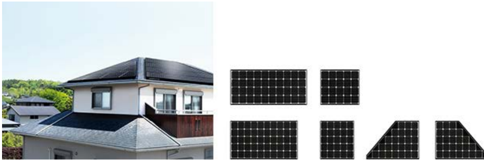
Multi Roof photovoltaic system
