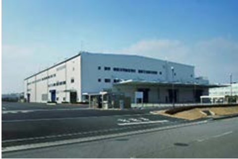
View of the plant
