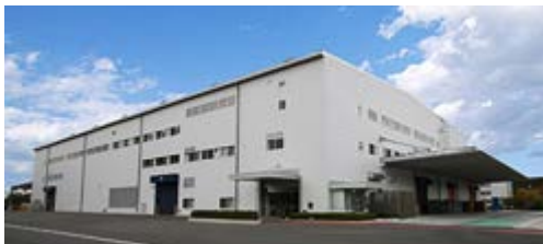
Green Cycle Systems Corporation. Japan's first large-scale, high-purity plastic recycling operation, turns plastic from end-of-lifecycle electrical appliances into new plastic material that can be reused in new home appliances.
