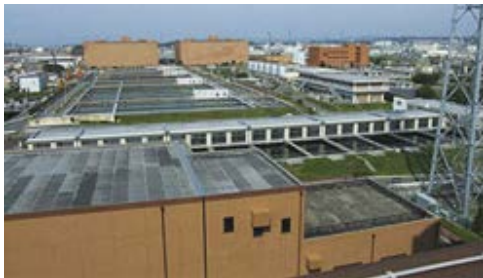
Murano Water Purification Plant
