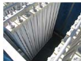
Microfilter module. One square pole contains 640 hollow filamentous membranes which absorb and filter impurities.
