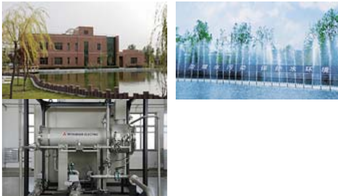
Qinghe Wastewater Treatment Plant and Mitsubishi Electric's ozone generator
