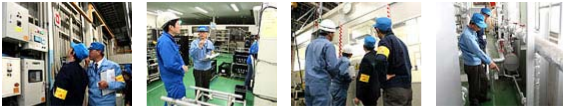
Energy conservation experts conducting inspections.
