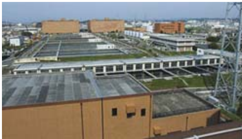
Murano Water Purification Plant
