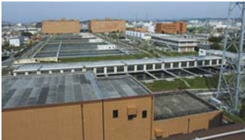
Murano Water Purification Plant
