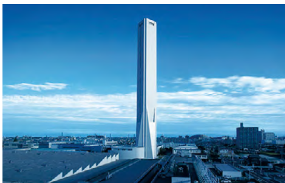
SOLAÉ elevator testing tower
