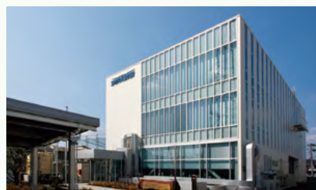
Shirasagi Denki Kogyo Co., Ltd. head office building
