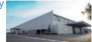
VI and VCB factory
